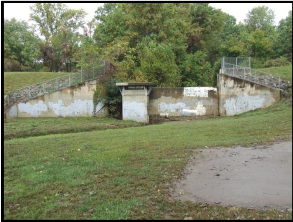
Stormwater dry pond at Victory Farm Park.
