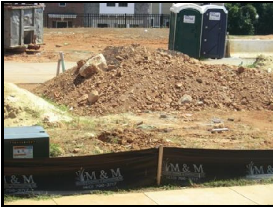
Construction site runoff controls to prevent soil loss and nutrient pollution
