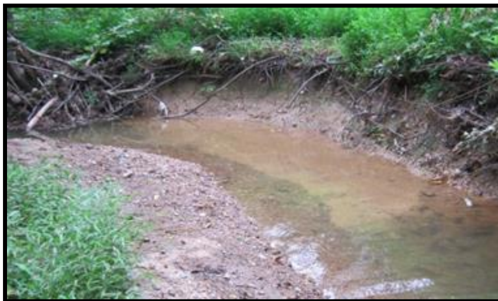
Stream bank erosion and woody in-stream debris at Malcolm King Park
