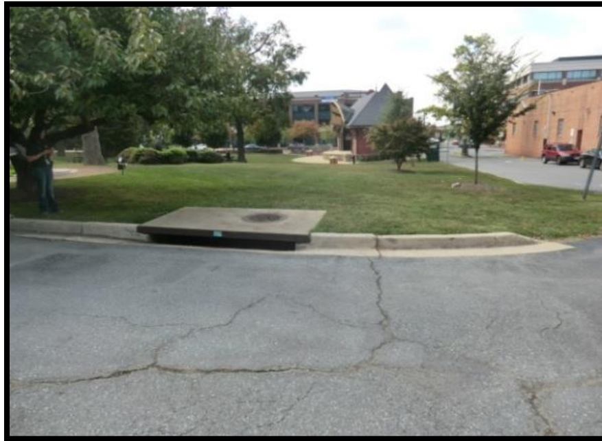
Existing stormwater drainage collection inlet for City Hall Parking lot.
