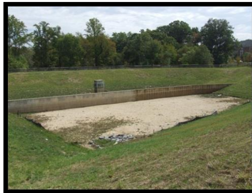
Sand filter located in Gaithersburg.
